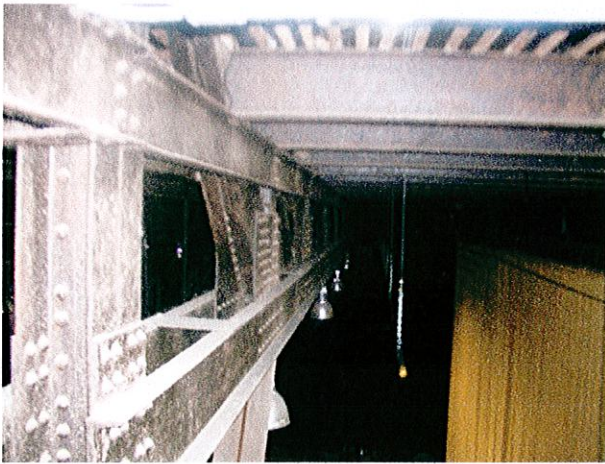
(a) A Hammerstein Stagehouse Truss
