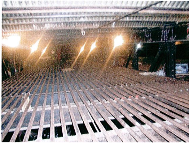
(a) Hammerstein Gridiron and Original Stagehouse Roof
