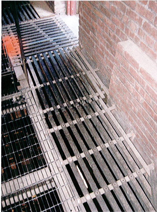
Figure 5 – Section of Original Slat Walking Surface of Gridiron (note modern bar grating to left)
